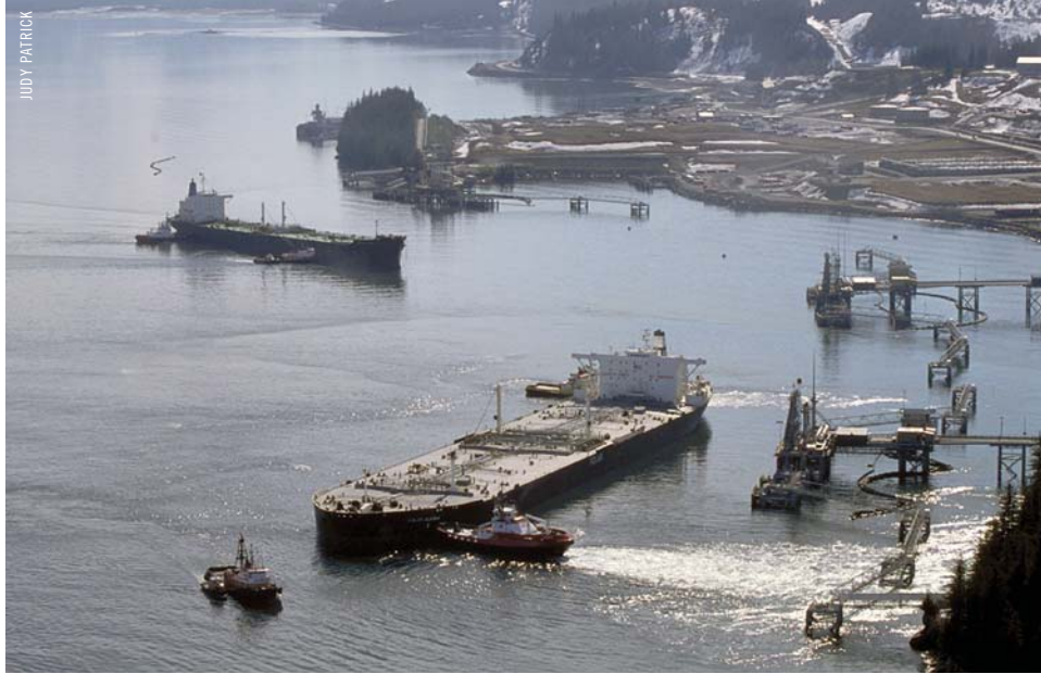
Oil tanker receiving terminal at Port of Valdez in Southcentral Alaska. The 800-mile trans-Alaska oil pipeline starts at Prudhoe Bay on the North Slope and terminates here.
